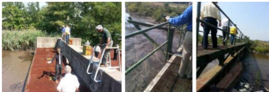
Figure 4-1: Physical Inspection of Existing Risk Reduction Infrastructure. Teams assigned by the New Jersey Department of Environmental Protection have endeavored to catalogue Superstorm Sandy’s impact on berms, tidal gates, and other existing risk-reduction infrastructure. Physical inspection is a key part of the State’s assessment of the current condition of measures to identify necessary repairs as well as opportunities to enhance existing measures to address future extreme weather events and maximize federal investment.
